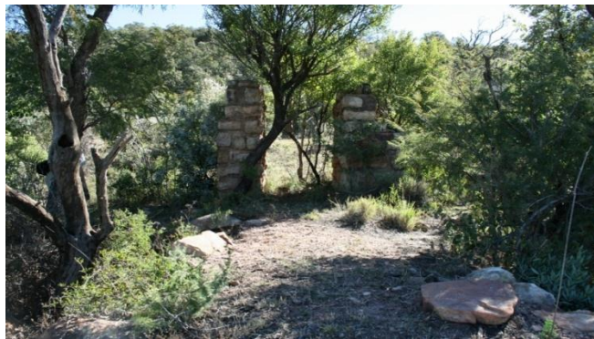
Figure 22. The foundation for a stamp mill at Nooitgedacht 508IQ. Milled sand was found next to this structure, as well as concrete anchoring posts pointing to the foundation hosting the stamp mill.
