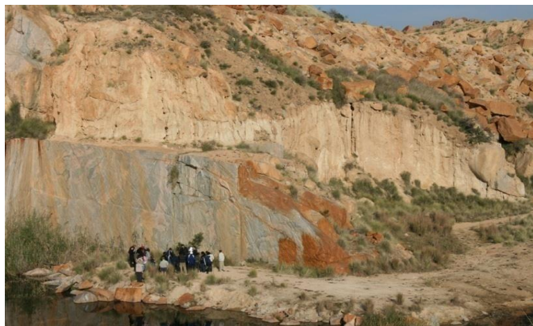
Figure 63. To the upper right of the group of people to the far right of the photograph unstable rock dumps and overburden at Leeukop Quarry GQ3 on Kopjeskraal 517IQ.
