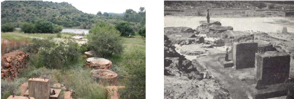
Figure 23. The remains of mining beneficiation infrastructure at the Great Western mine. The rectangular cement blocks in the foreground were part of the foundation of a stamp battery, whilst the rounded, cylindrical structures were the bases for cyanide leaching bins. Compare the photograph at the right (from Kriel & Germishuys, 1957) with the one taken in 2010 (fifty years later).
