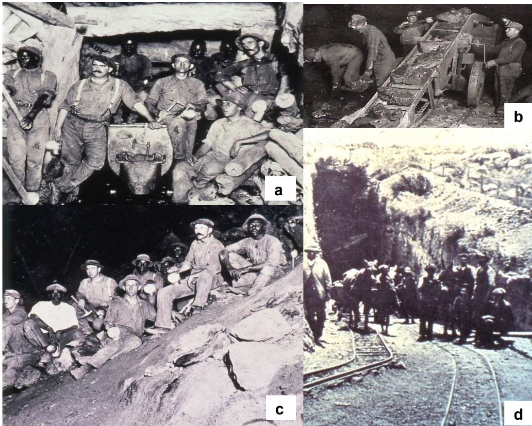
Figure 8 a-d. Historic mining photographs (courtesy Ben van Wyk, Extract Training Pty Ltd., photographer unknown). See text for more detailed description. Figure 8a shows some equipment, the wooden support and the poor initial safety standards where hard hats were optional. In Figure 8b a hand operated conveyance system running on tracks can be seen. An inclined stope and the use of carbide lamps are visible in Figure 8c. The use of mules to convey hoppers is seen in Figure 8d.
