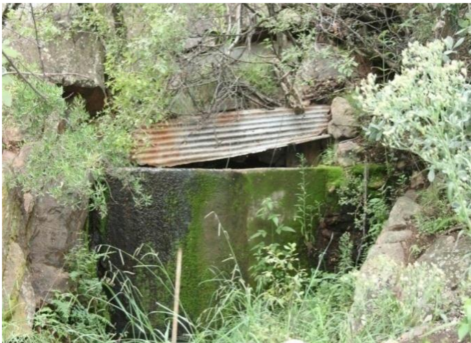
Figure 71. Mine adit KF1 at Koedoesfontein 478IQ partially closed for water extraction.
