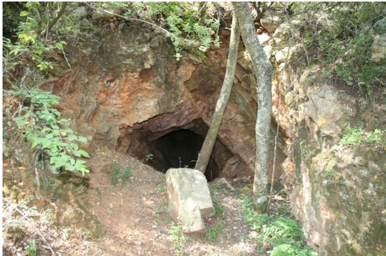
Figure 60. An adit QB13 on Buffelskloof 511 IQ with bad overhang at the entrance.
