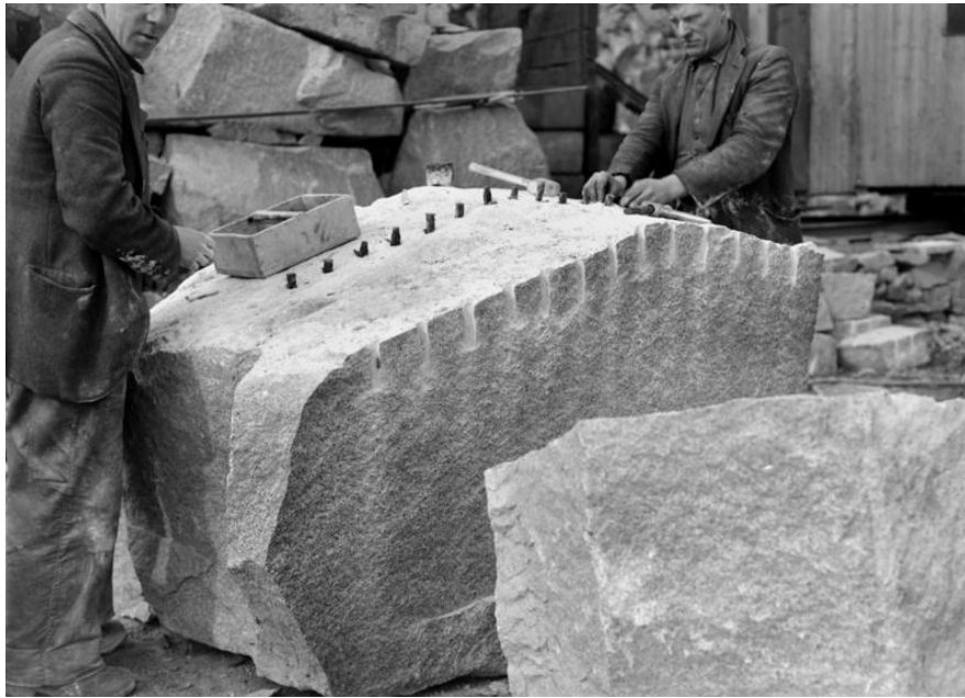
Figure 42. A historic photograph from Silver Grey Quarry, Creetown. Kirkcudbrightshire. Two quarrymen can be seen inserting the 'plug and feathers' into a large granite block. A recently separated block can be seen in the foreground. This photograph was copied from the Drystone garden website (Drystone, 2012)
