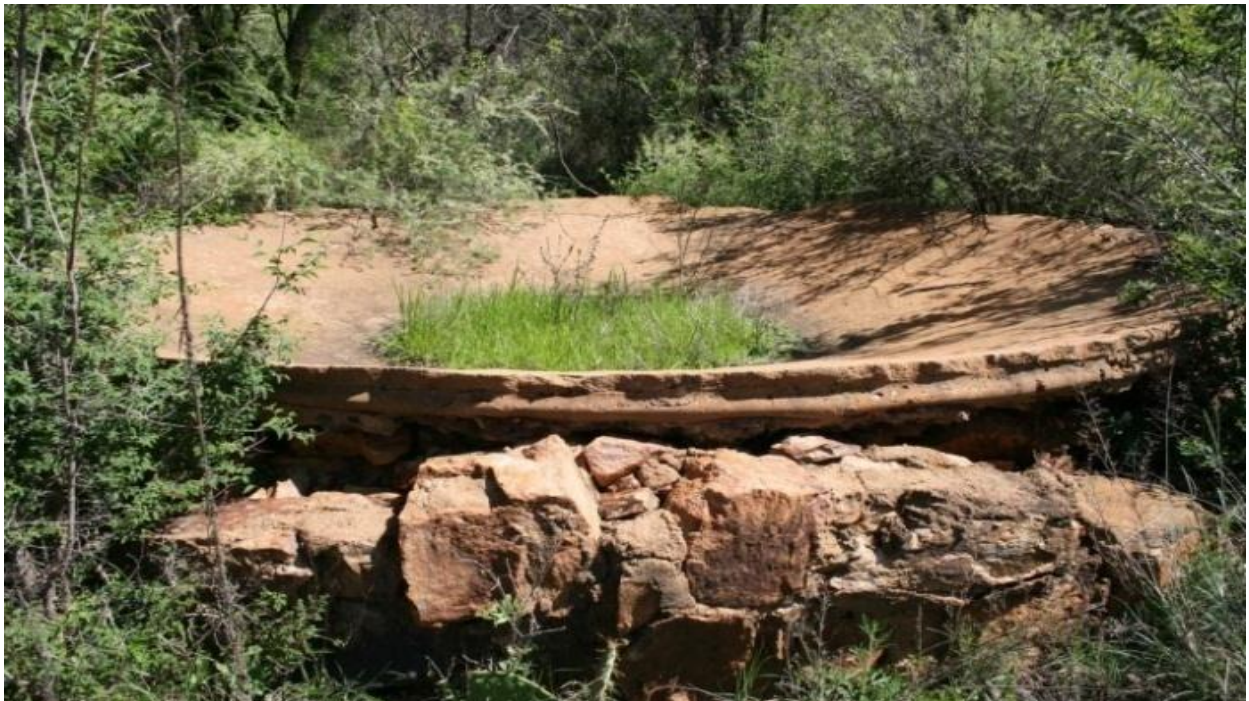
Figure 56. Similar cyanide bin foundations at the Colin Voi mine, N1 on the farm Nooitgedacht 89.
