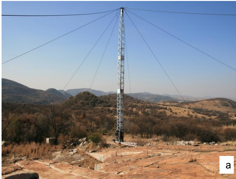
Figure 52. (a) The steel pivot structure at Spitzkop Quarry, GQ13, with the stabilizing cables still in place. (b) An old photograph of possibly the same quarry when in operation. This photograph was copied from the Marlin website (2012).
