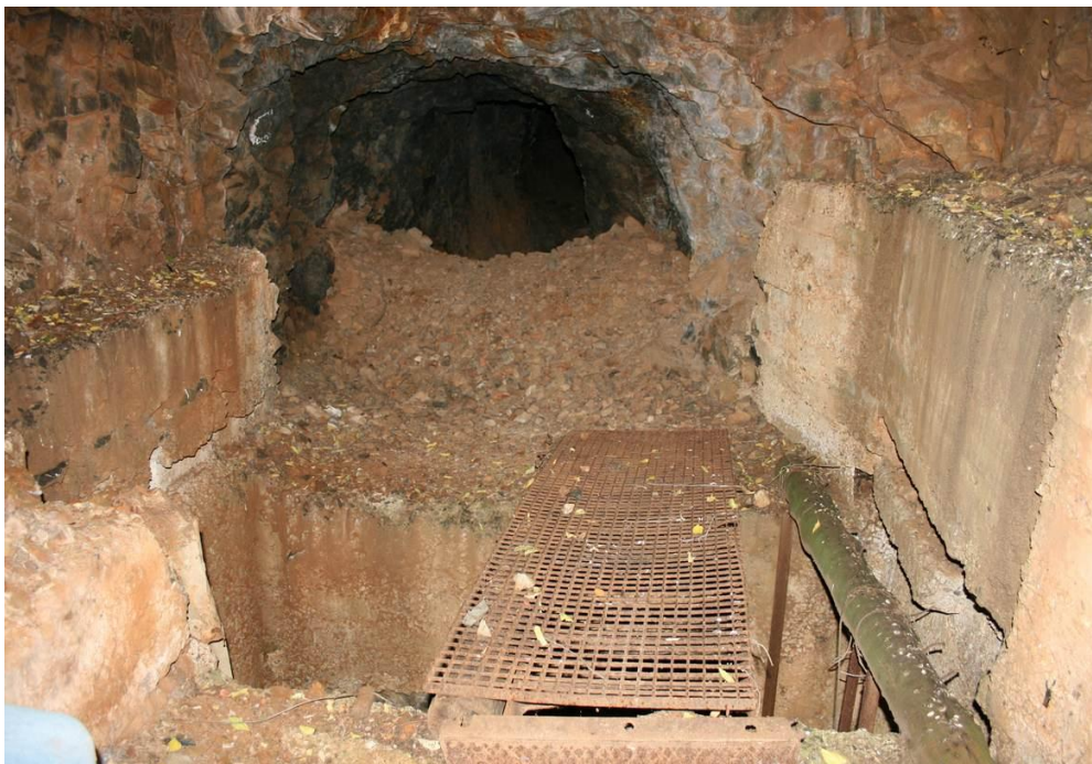
Figure 28. Underground infrastructure covering a water filled shaft and leading to an unventilated end at Rebokkop 290.
