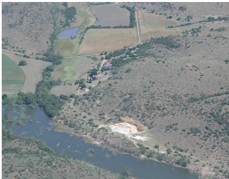
Figure 73. The erosion of tailings slimes into the Vaal River at Great Western Mine, E1, Elandslaagte 28.
