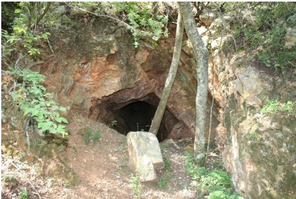
Figure 14. Adit, B9, on the eastern portion of Buffelskloof 511IQ with dangerous overhang at the entrance.
