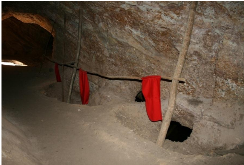
Figure 59. An adit at R19, Rooderand 510 IQ where the stoping from the bottom level holed into the reef drive. The red flags were used in an attempt to warn visitors of the danger when walking past the site after abseiling down from a raise holed to surface (where sunlight enters to the left hand side of the picture).
