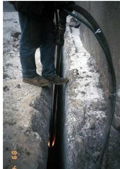
Figure 38. Thermal lance cutting a slot in granite. This photograph was copied from the Techcorr website (Techcorr, 2012).
