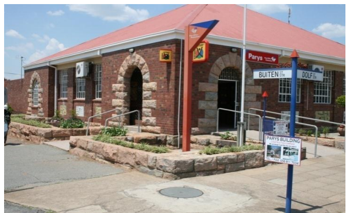
Figure 36. Granite blocks used in the construction of the post office, Parys.
