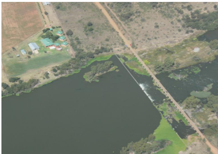
Figure 67. Schoemansdrif in 2007, with the irrigation dam wall seen on the left hand side of the bridge (note also the presence of the hyacinths and eucalyptus trees).
