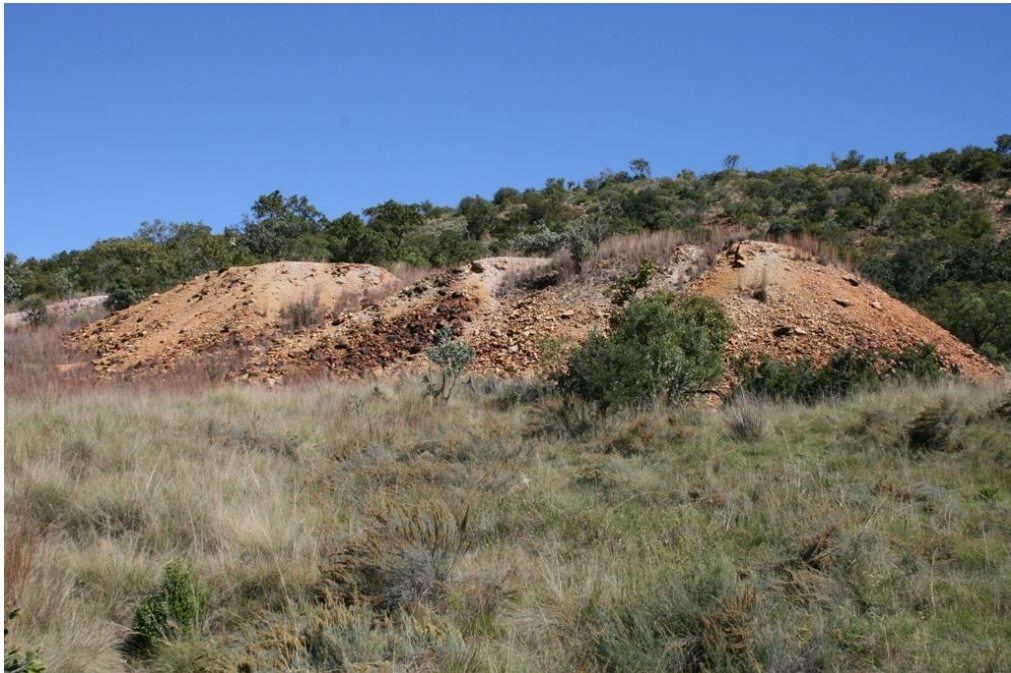
Figure 17. Mine workings, visible from the road (between Potchefstroom and Venterskroon) at Rooderand 510 IQ. The colour difference is due to weathering of pyrite present in the mined material.
