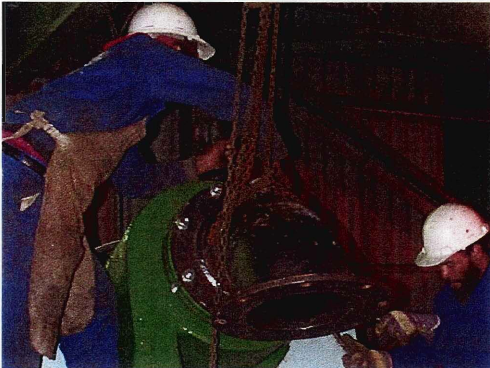
Photo's 12 & 13: Installation of 510 mm Multotec cyclone at Koingnaas Main Plant
