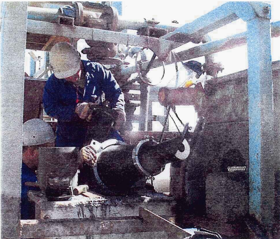
Photo 4: Installation of 250 mm PU cyclone at Koningnaas Prospect Plant
