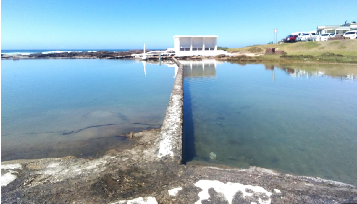
Fig. II: Site 195, 210 & 510. Tidal pool at Kidd's beach with a new pool that formed next to the pool wall.
