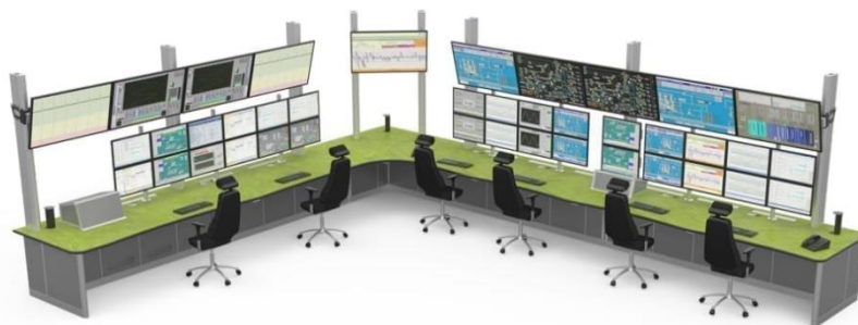
Figure 10: Control room used as a central point where all operations can be monitored and controlled 6
