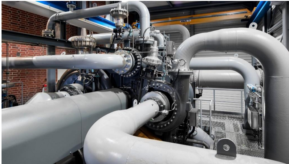
Figure 9: Multistage compressor with pipelines used to transport fluid to end users 5
