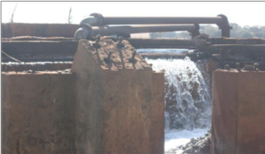
Figure 7-4 Decanting ventilation shaft near Tweelopiespruit
