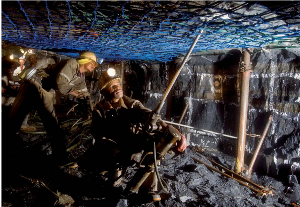
Figure 4 – Pneumatic rock drills in operation 6
