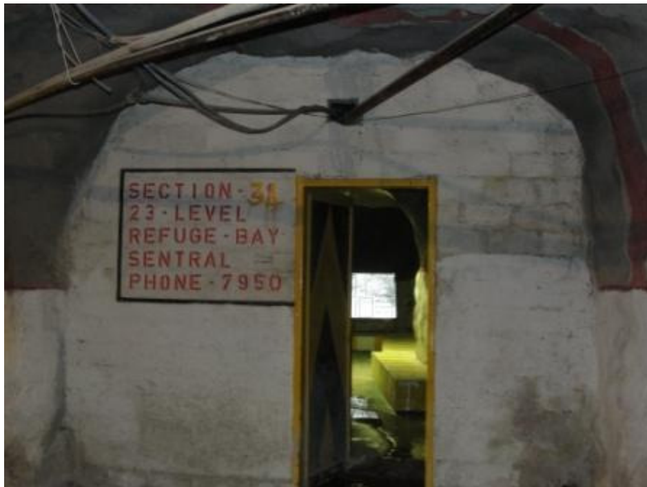
Figure 7 – Underground refuge bay 9
