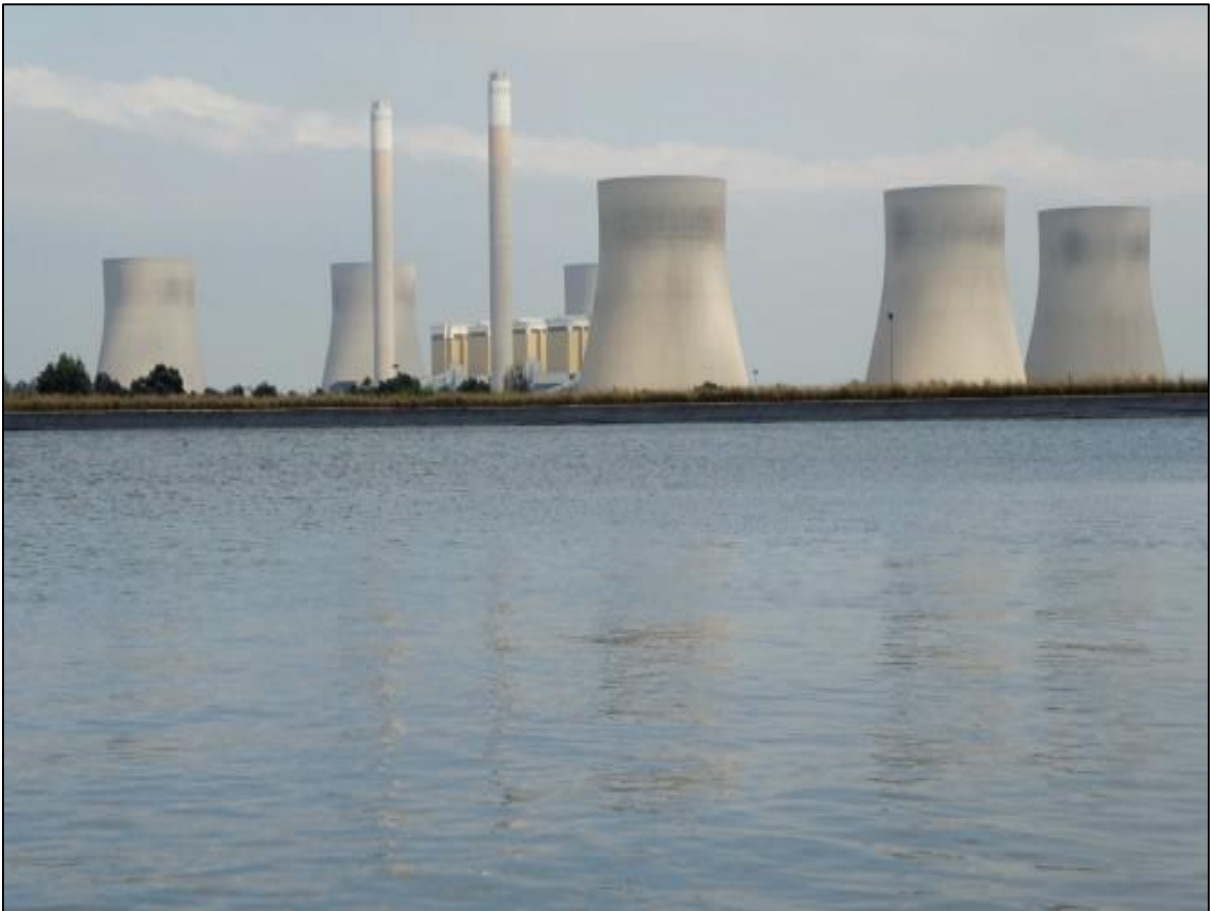
Power station with water supply dam in foreground 1
