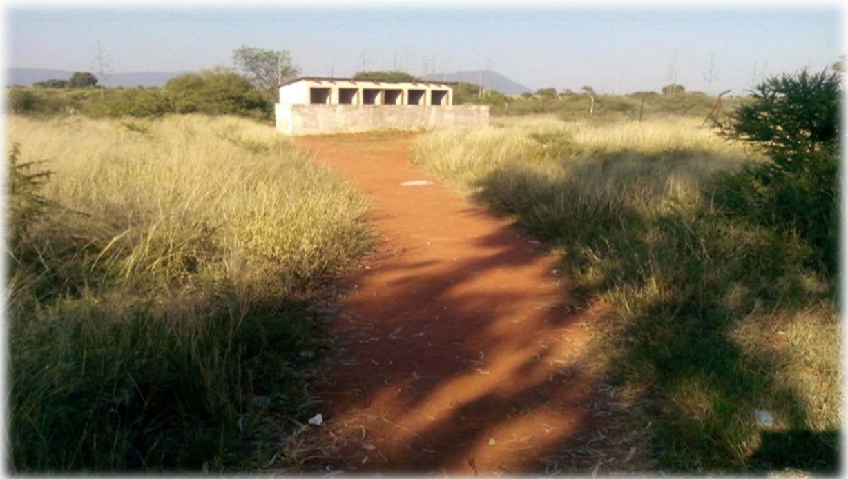
Figure 5-9 Toilet structures for learners (boys) with extremely overgrown surroundings
