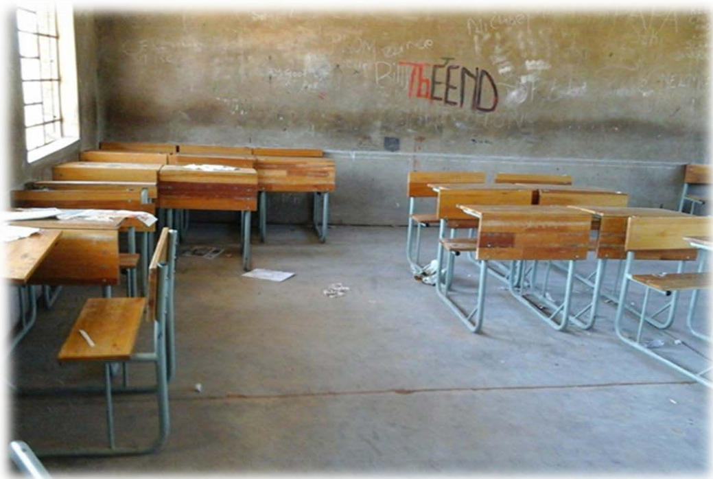
Figure 5-5 Condition of one of the classrooms
