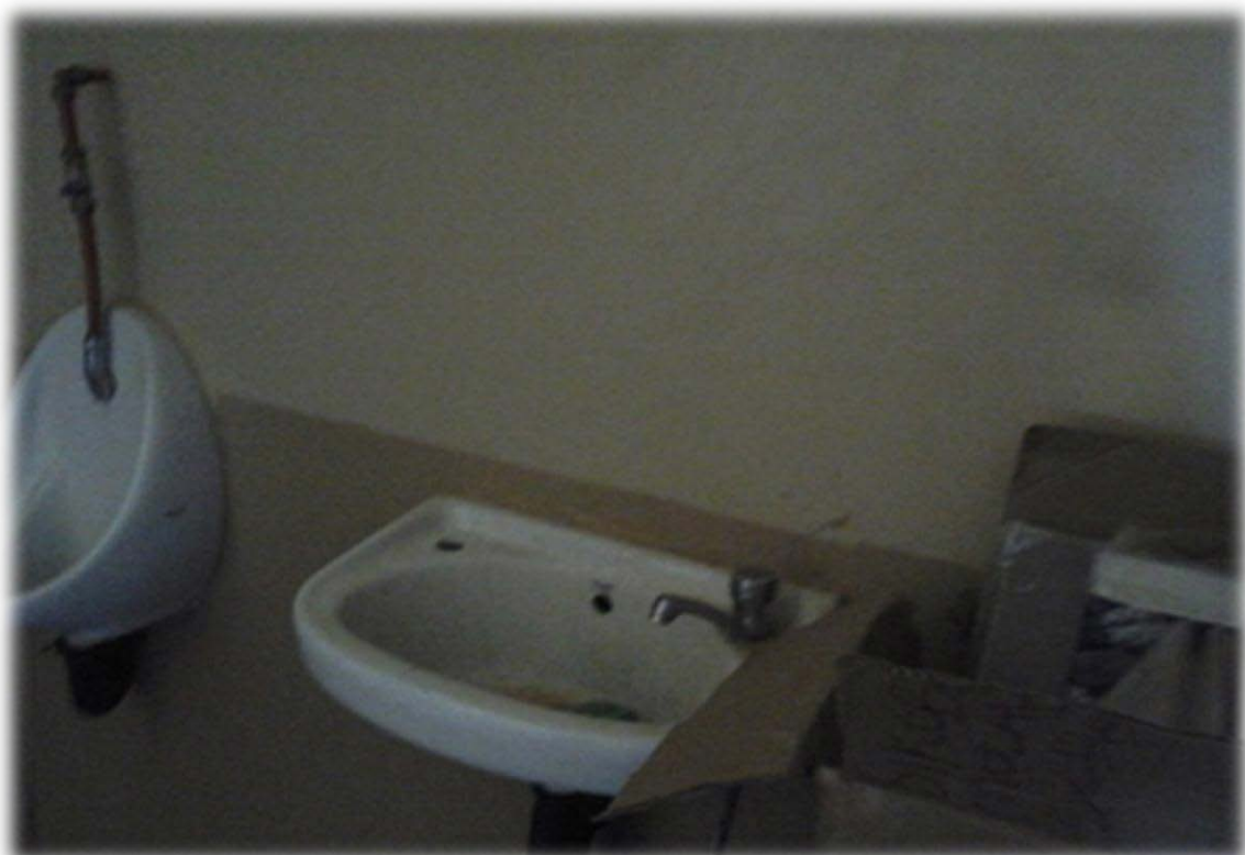
Figure 5-2 Wash basins and toilets in the building near the entrance gate
