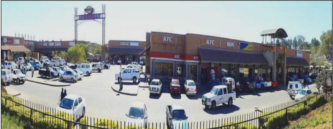
Figure 8-5: Hubveni Shopping Centre
