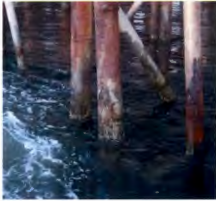
Figure 1.1: Waterline corrosion
