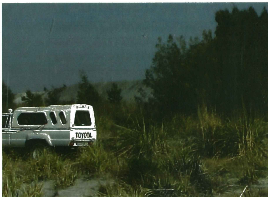
FIGURE 17: ONE OF THE DENSELY VEGETATED AREAS OF THE TAILINGS DAM.
