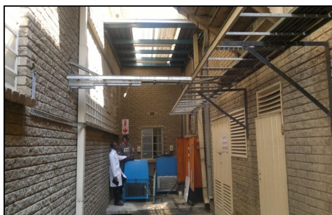
Figure 25 Air compressors in confined space
