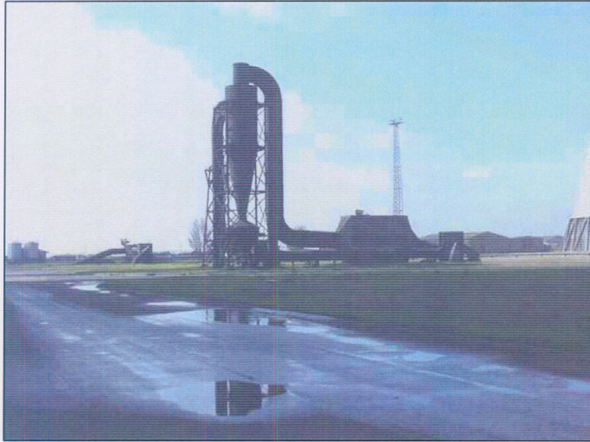
Figure 4: The FCP at Hendrina Power Station.
