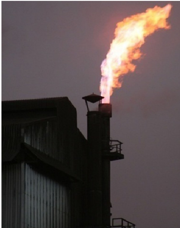
Fig. 1—A typical CO-rich off-gas flare on top a closed FeCr SAF stack.
