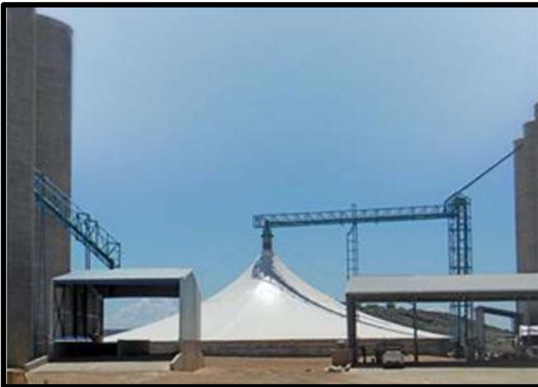
Figure 2.11 – Tent silo complex
