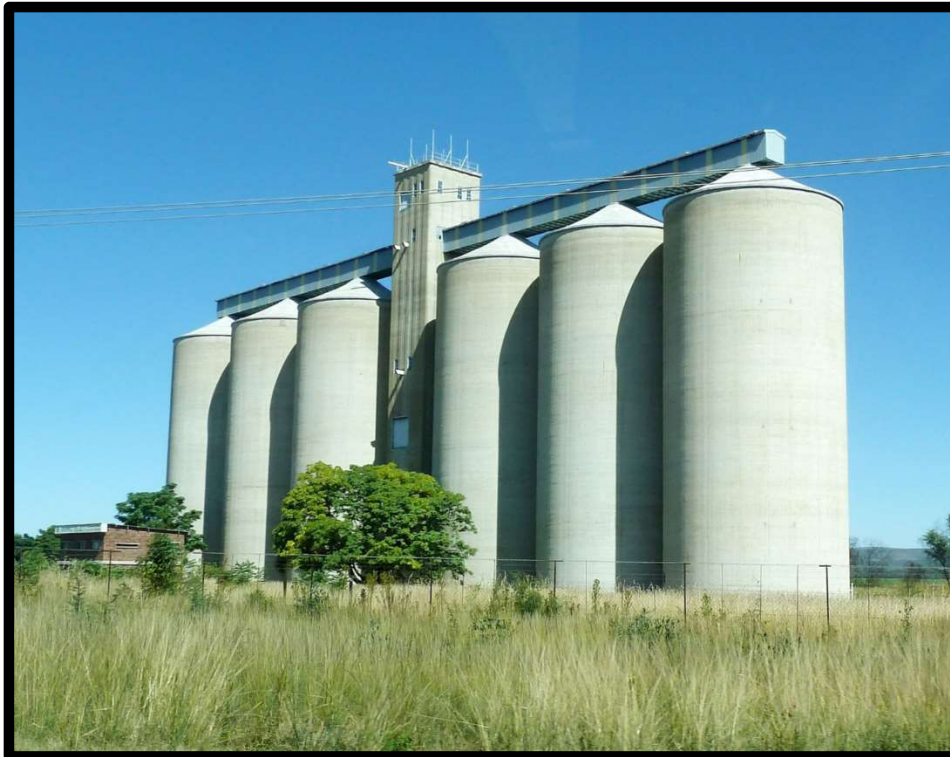
Figure 2.5 - Concrete grain silos – Vaalwater, Limpopo
