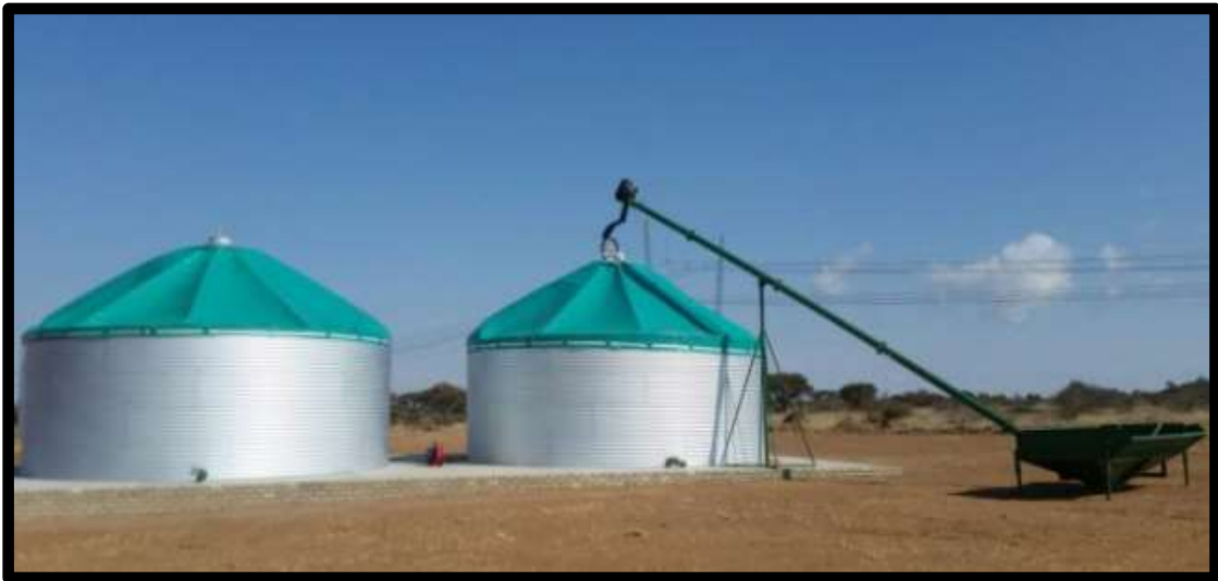
Figure 2.14 – Grain dam - Zinc
