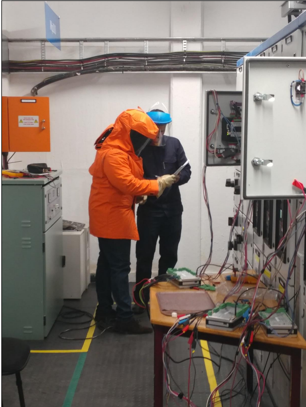
Figure 3: Synchronizing Generator to LV Network
