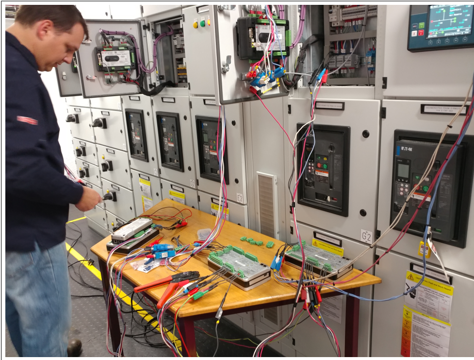
Figure 4.2: Installation of a Vecto II and Impedo Duo metering instruments
