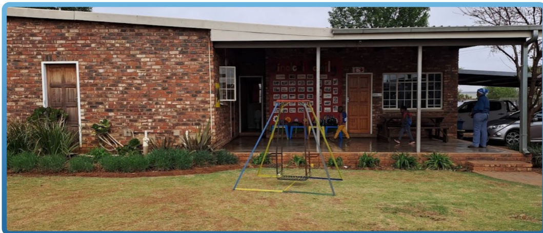
Photograph 6-6: Structure of C3.
