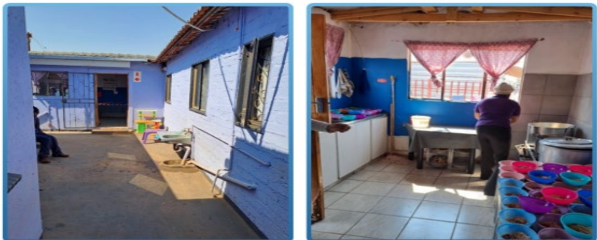
Photograph 6-2: Structure of C1.
