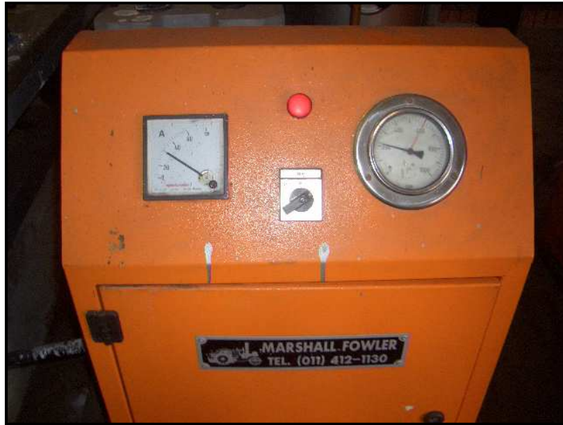
Figure D.1.2: Electrode boiler rated at 60 kg/h saturated steam at 600 kPa pressure
