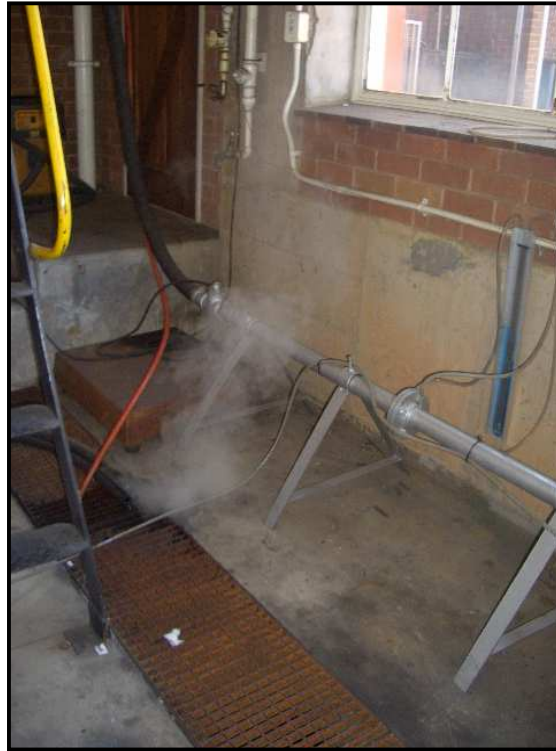
Figure D.1.11: Airflow orifice plate and manometer
