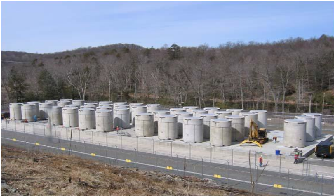
Figure 2-6: Connecticut Yankee dry cask storage facility (Connecticut Yankee, 2019)
