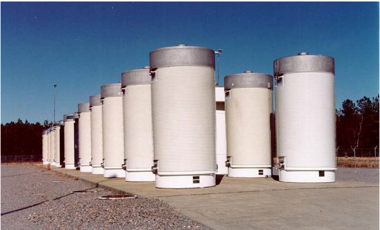
Figure 2-12: Example of metal cask stored on an open reinforced concrete storage pad open to the environment at Surry power station, Virginia USA (Skrzyppek & Kim, 2015):
