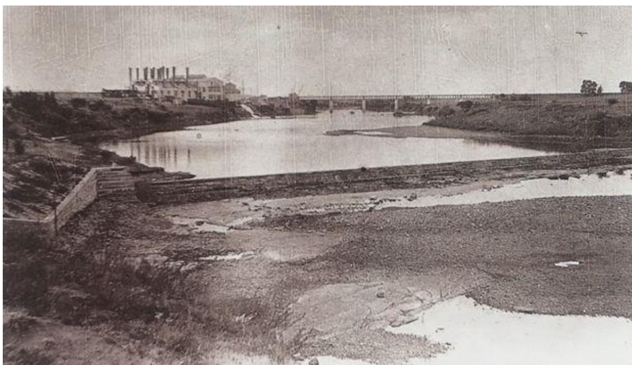
Figure 67: Vereeniging Power Station – drought interrupted flow of Vaal River [3]
