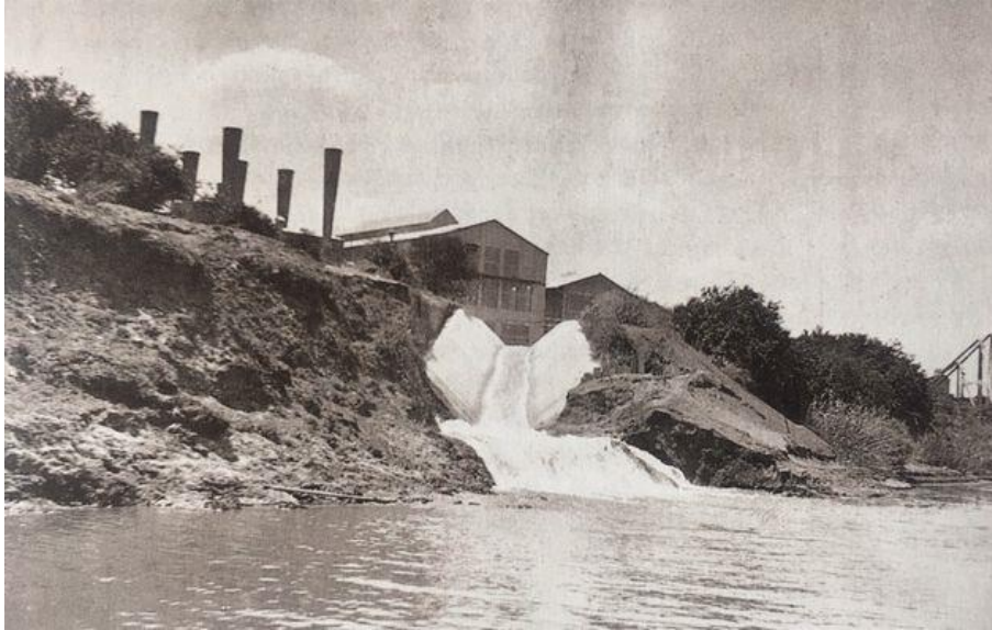
Figure 66: Vereeniging Power Station (1912) – warm water returns into the Vaal River [3]
