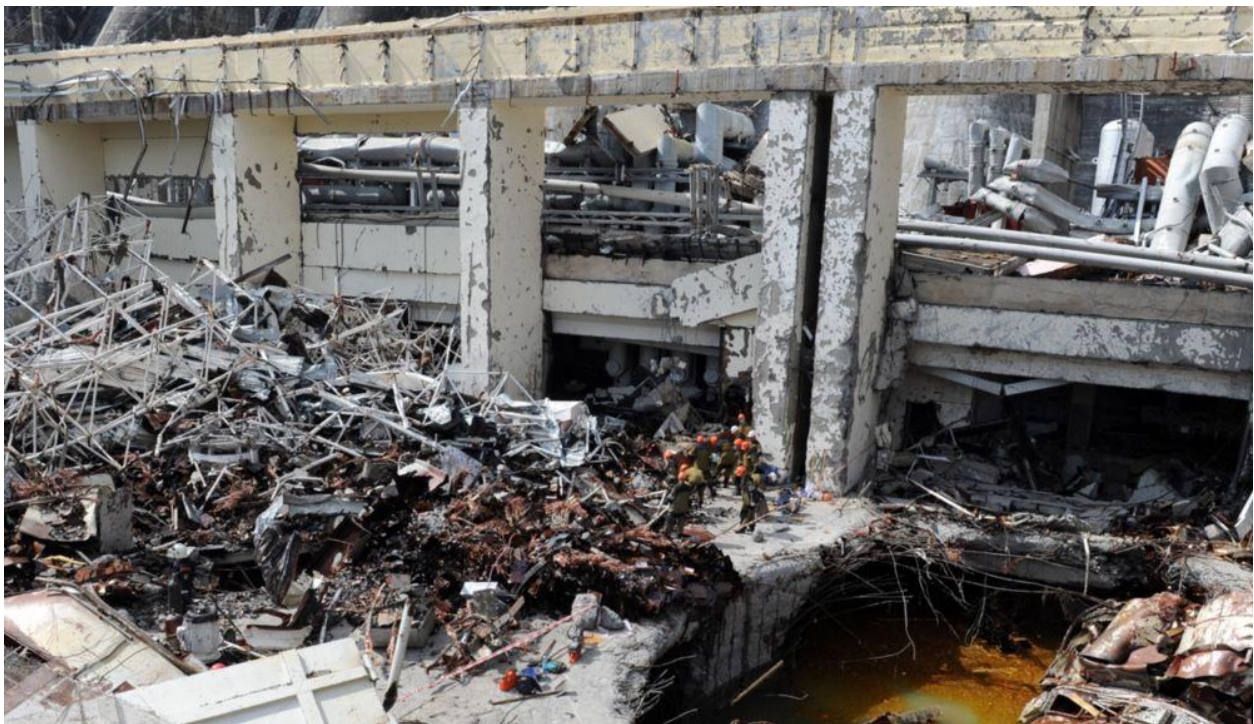
Figure 54: Catastrophic flooding failure of Sayano-Shushenskaya Hydroelectric Power Station [165]
