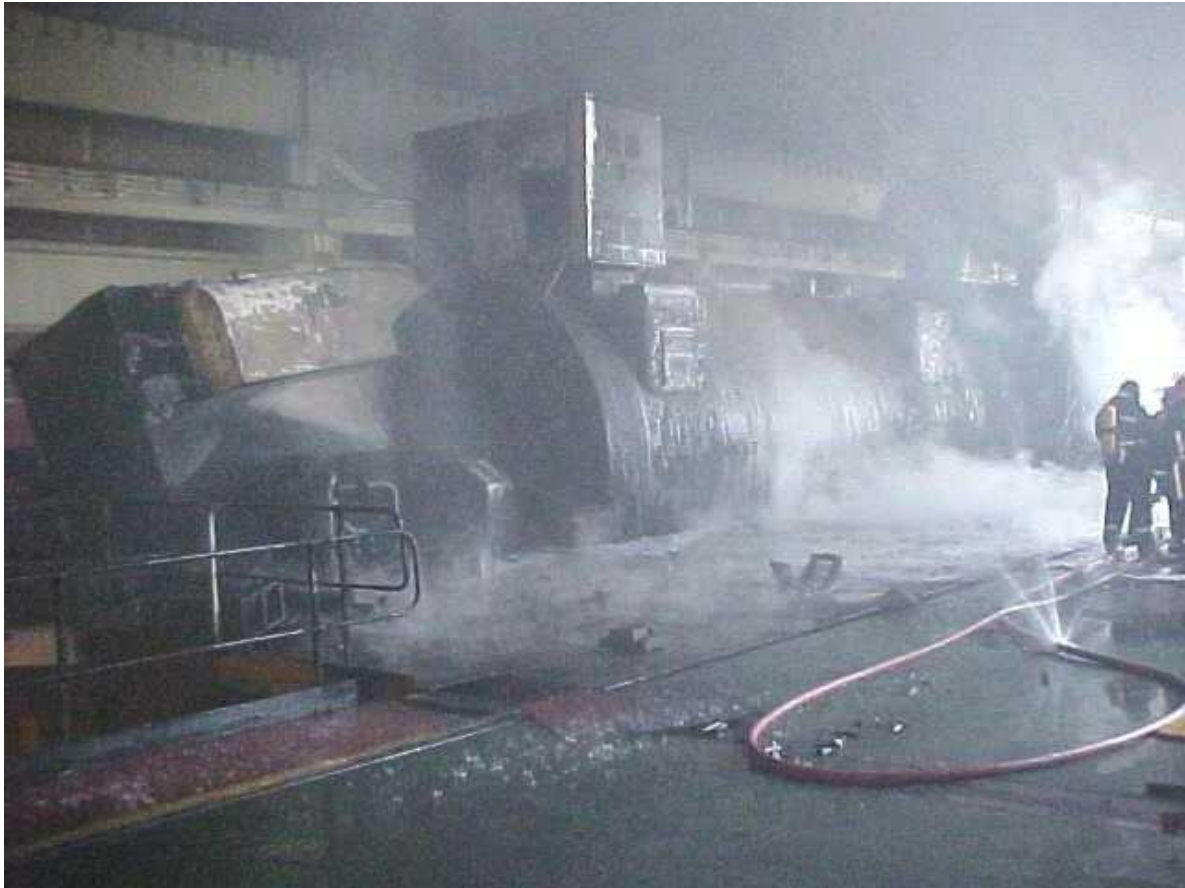
Figure 56: Duvha Power Station following a catastrophic turbine over-speed failure in 2011 [168]
