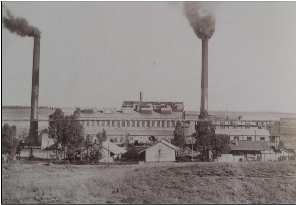
Figure 4: Brakpan Power Station [3]
