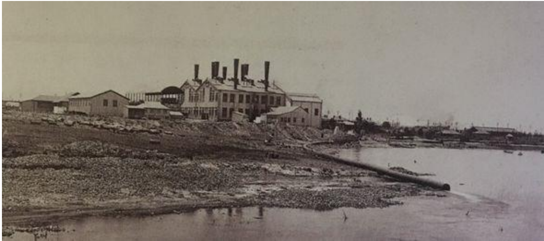
Figure 64: Simmerpan Power Station (1912) – water return in foreground (40 MW installed) [2]
