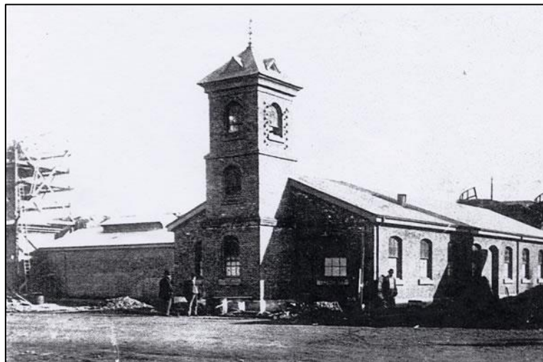
Figure 2: The Table Bay Harbour Electric Light Works – the first central power station in SA [2]
