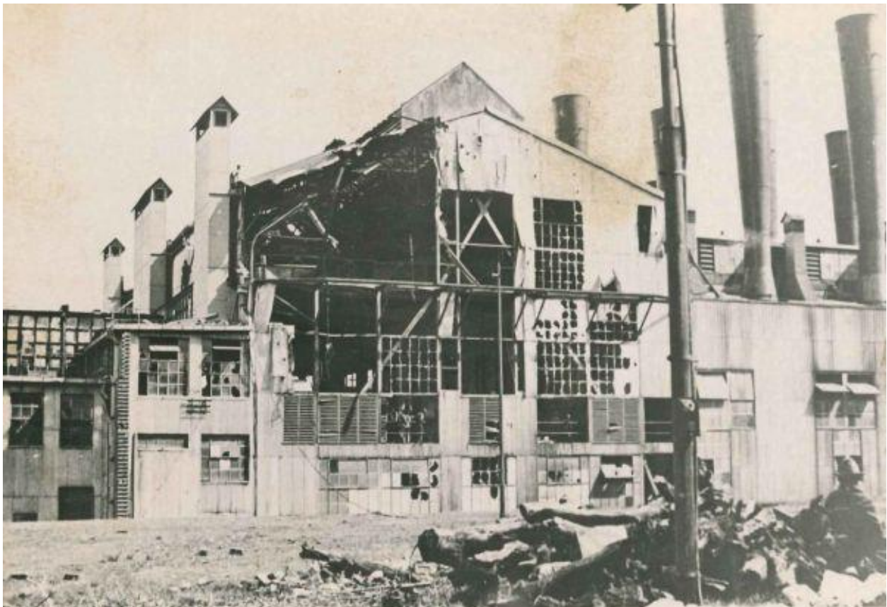
Figure 55: Vereeniging Power Station following a catastrophic failure in 1925 [2]
