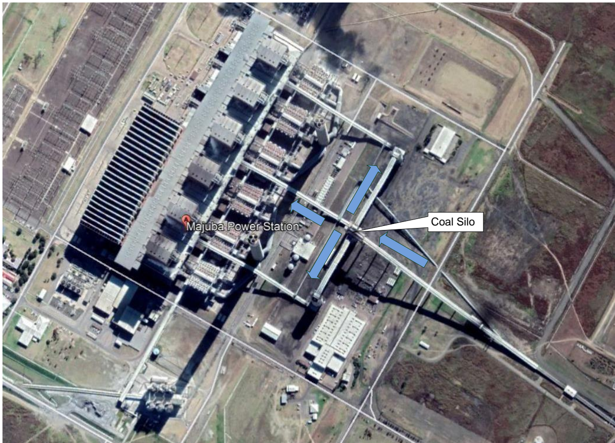
Figure 60: Majuba Power Station coal supply conveyor system [170]
