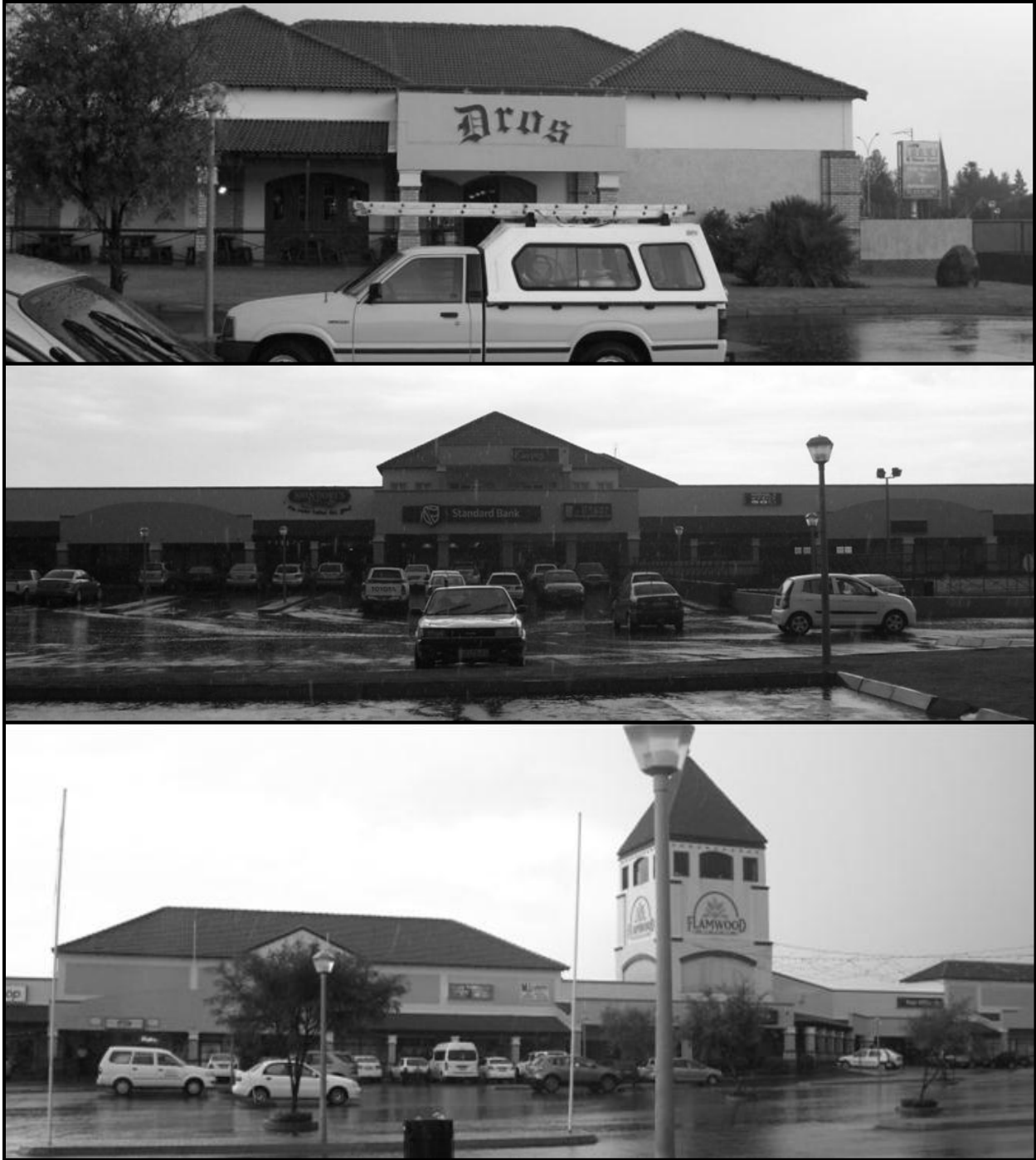
Figure 15: Flamwood Walk Shopping Centre
