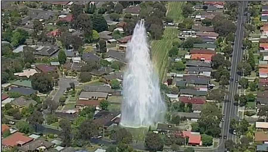
Figure 28: Example of a large pipeline burst [50].
