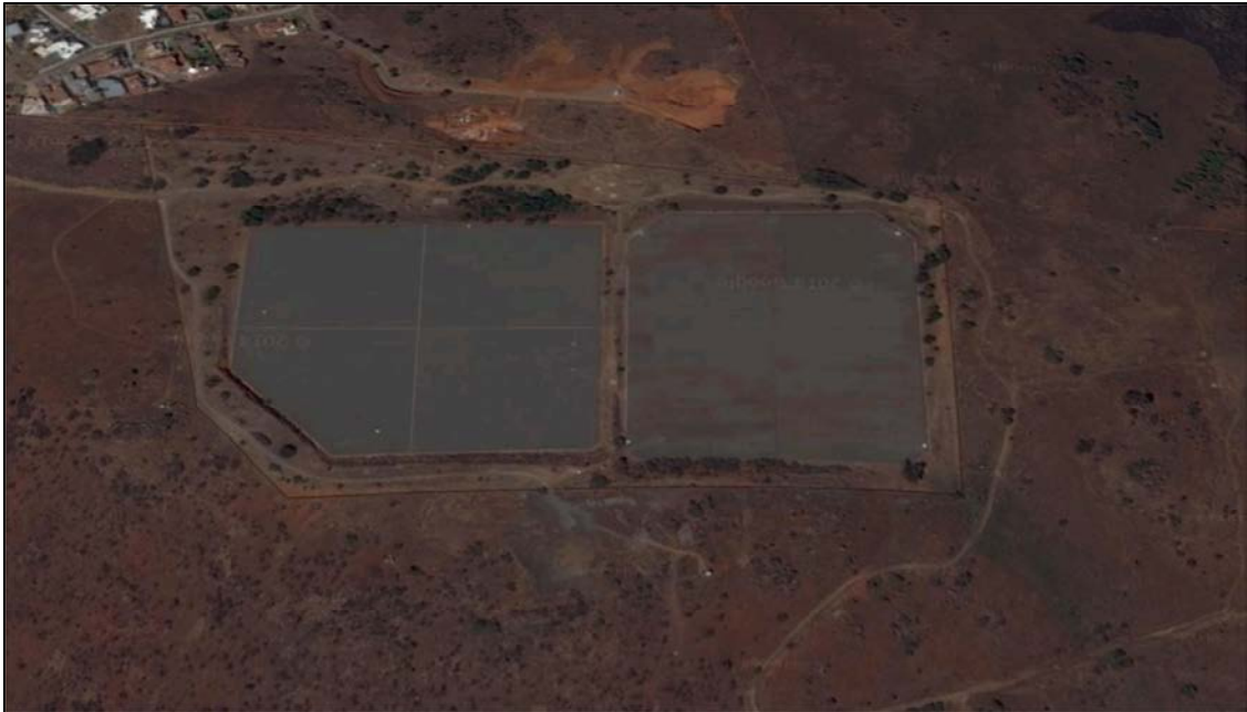
Figure 14: Aerial view of downstream reservoirs [22]
