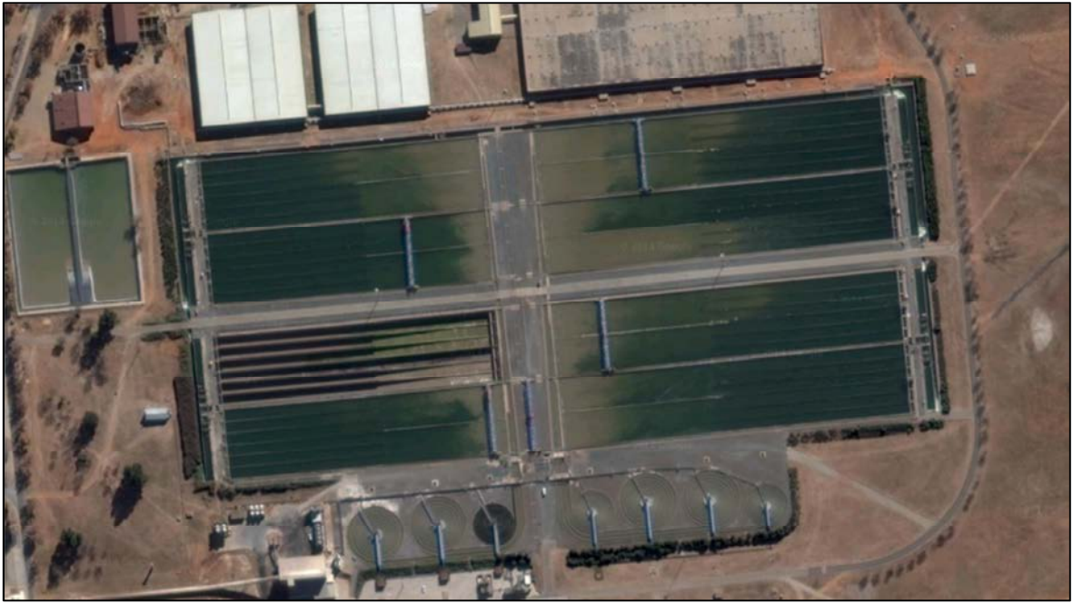
Figure 16: Aerial view of a clarifier [24]
