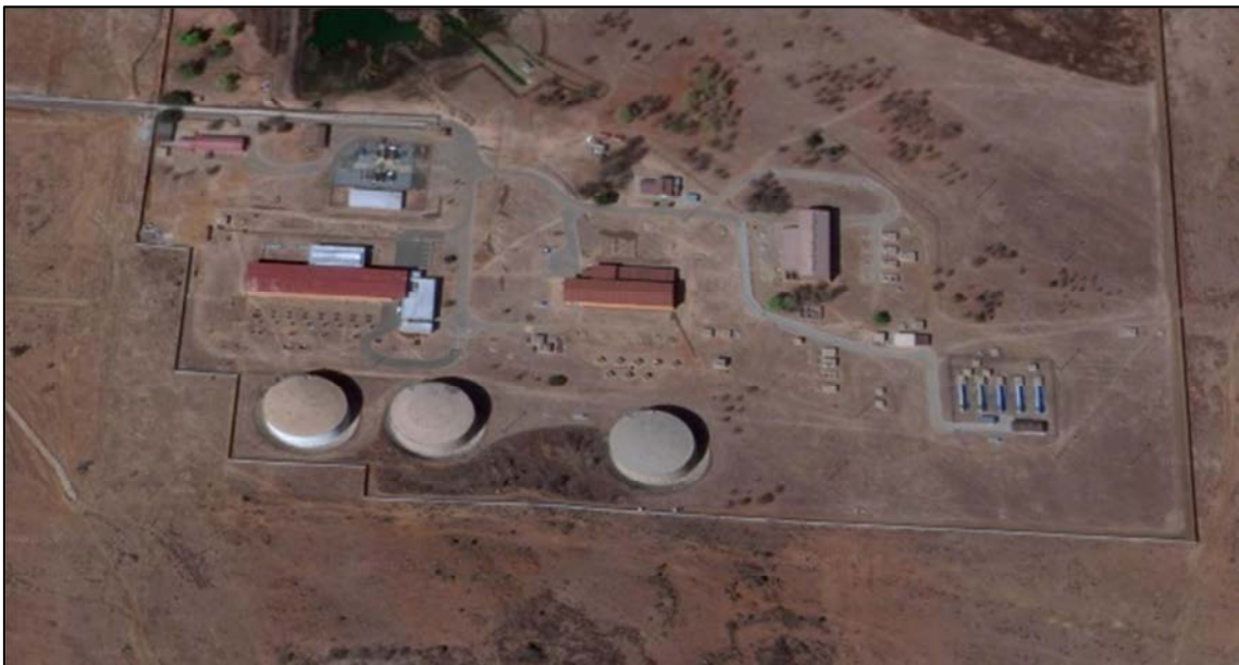
Figure 13: Aerial view of balancing reservoirs [20]
