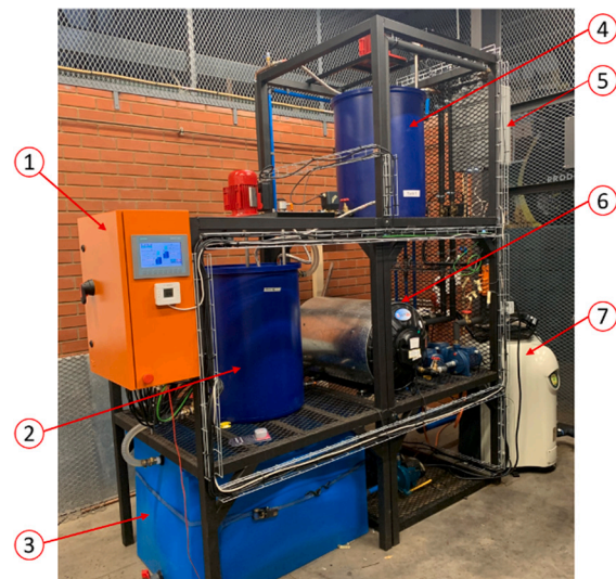
Fig. 3. Constructed pilot plant of the process in Fig. 2.
