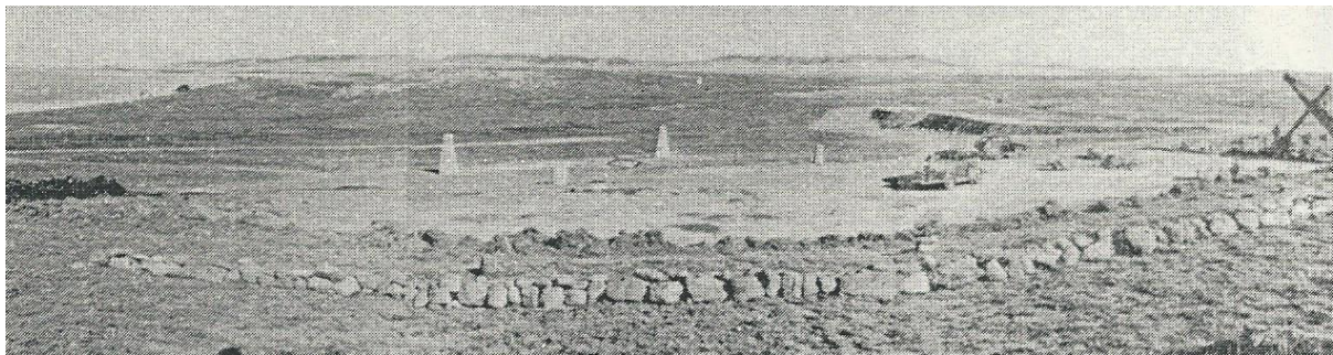
SINKING OF SHAFT NUMBER TWO AT WEST DRIEFONTEIN
