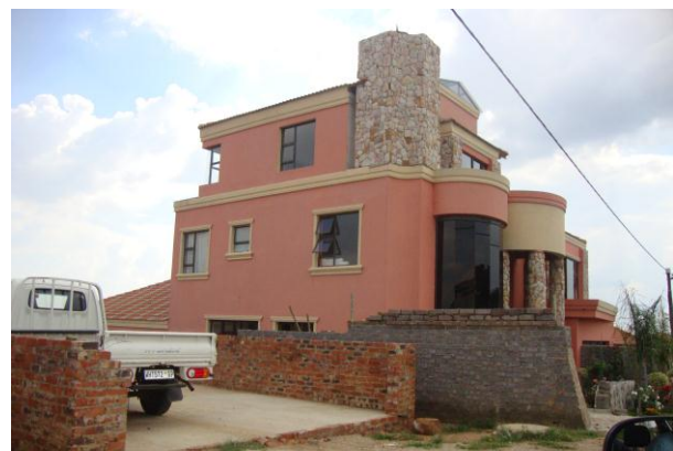
Figure 42: An expensive bonded home in Cosmo City
