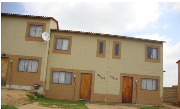
Figure 45: A double storey semi-detached unit in Olievenhoutbosch
