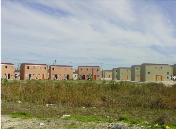
Figure 50: A typical image of units delivered in the N2 Gateway Project
