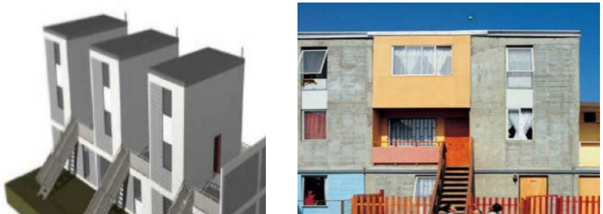
Figure 54: An initial building structure as received by tenants and the manner in which units can be extended by filling the space between starter units
