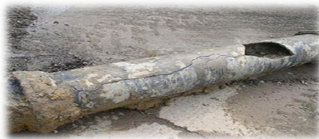
Figure 2-18: Damaged column caused by water hammer [47]
