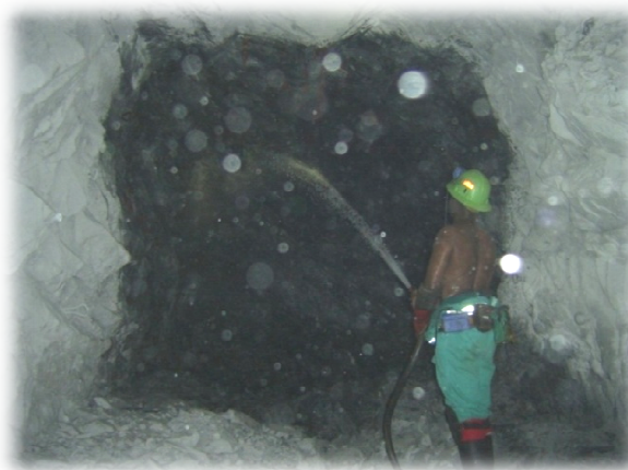
Figure 2-8: Water used to cool the rock surface
