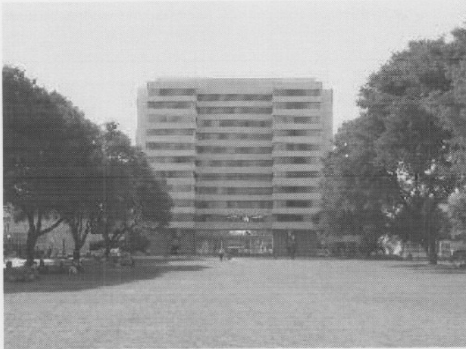
Figure 9-1: Front view of the Engineering Tower
