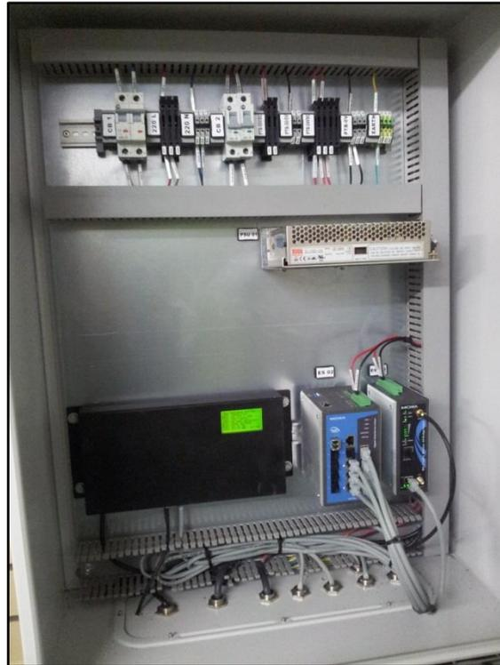
**Figure 41:** GSM Router installed at Rietfontein pump station
