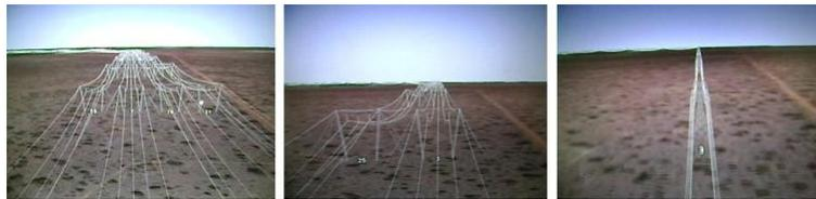
Figure 1.1: Effect of multiple power line circuits in a single corridor. The corridors transmit equivalent electrical power. Left: A corridor with four  $400kV$  circuits. Middle: A corridor with two  $765kV$  circuits. Right: A corridor with one  $765kV$  double circuit.
