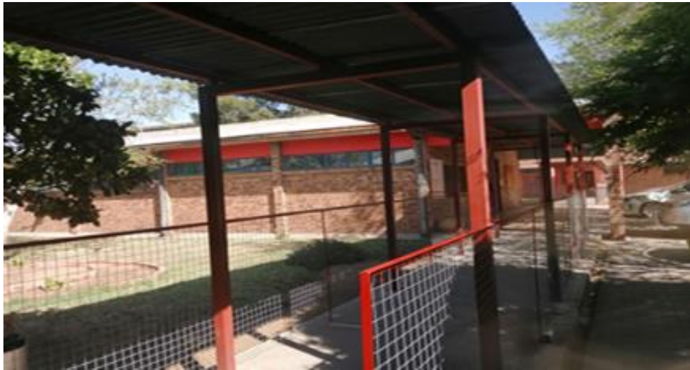
Figure 4.5: A channelling walkway for visitors to administration building
