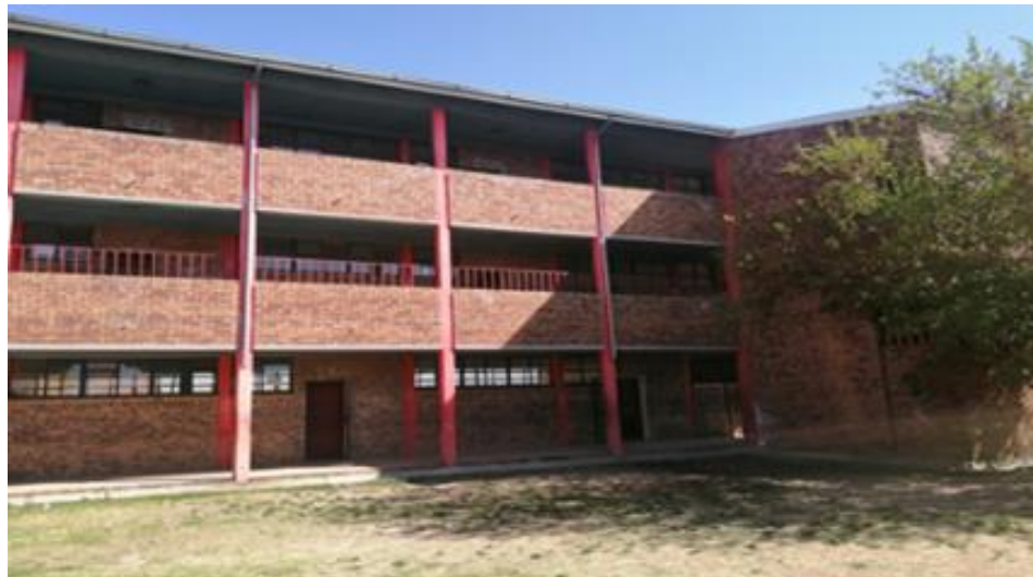
Figure 4.2: The three-story building type school
