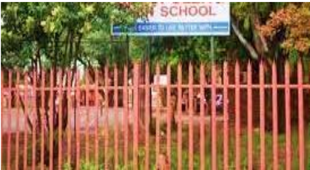
Figure 4.3: Sturdy metal palisade perimeter fencing at Kukhanya Secondary School
