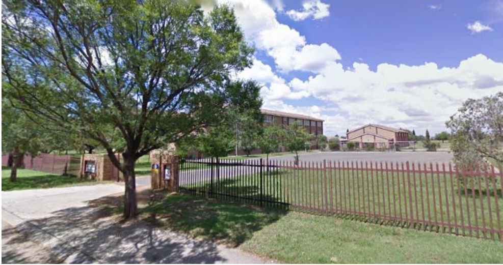
Figure 4.4: Sturdy metal palisade perimeter fencing at Ikatleleng Secondary Schools
