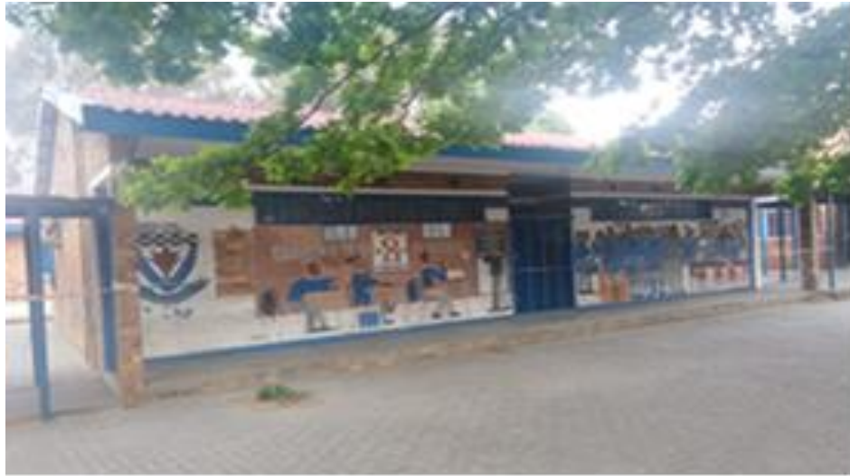
Figure 4.1: A single story building type school
