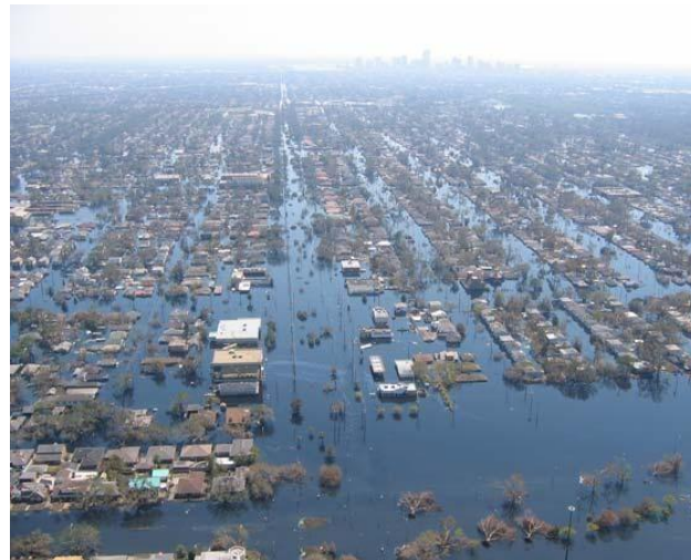
Figure 5.3 Hurricane Katrina damage (Image credit: NWS/Lieut. Commander Mark Moran, NOAA Corps, NMAO/AOC)
