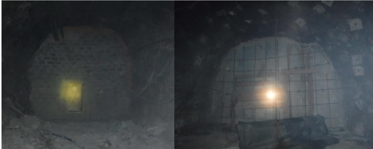
Figure 1-10: Typical ventilation seals 4
