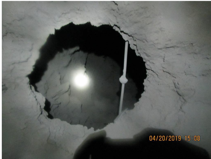
Figure I-5: Hole blasted in the wall
