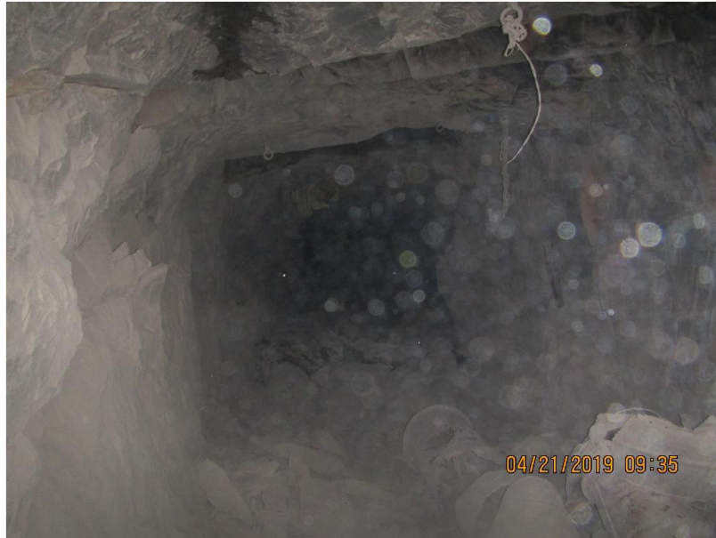
Figure I-6: Wall entirely removed
