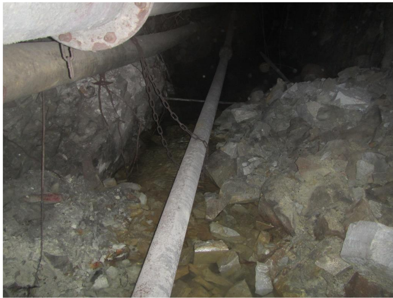
Figure I-1: Condition of airways in Zone 2
