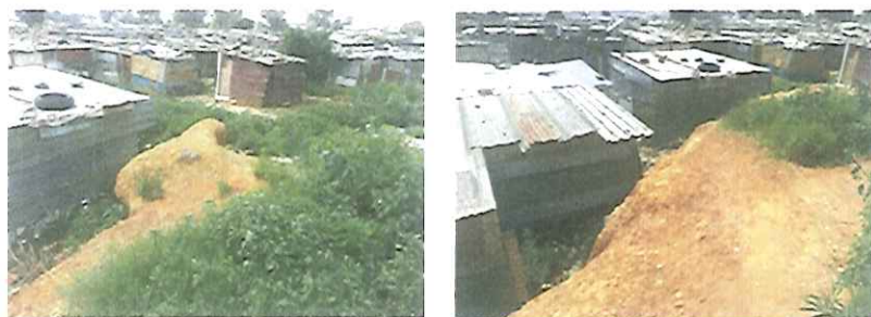
Figure 8: Informal houses at a distance of less than one meter from the TSF
