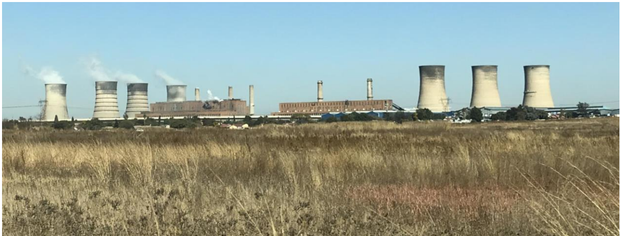
A Coal-Fired Power Station
