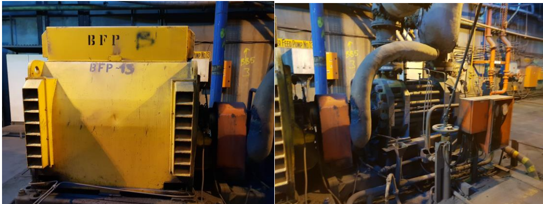
Figure A-7: Multi-stage electric feed pump
