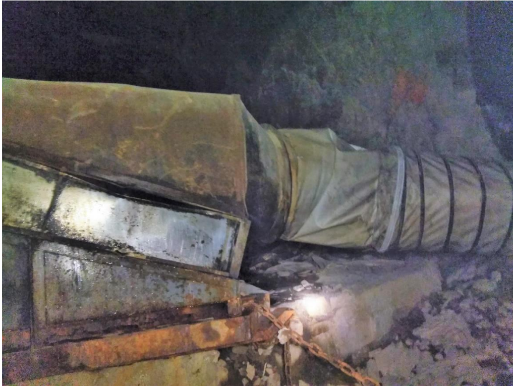
Figure 3-3: A 500-kW rated cooling coil installed underground xxi
