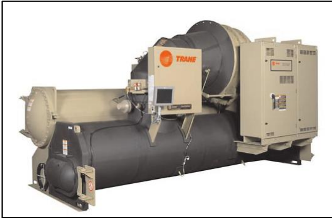
Figure 18: Vapour-compression chiller [30]
