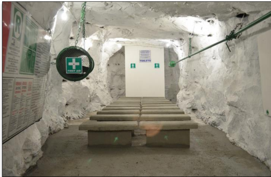
Figure 11: Underground refuge bay [51]
