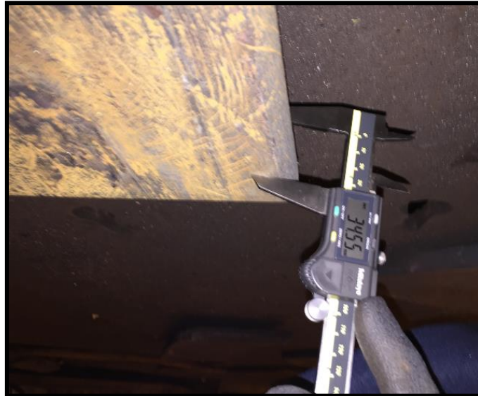
Figure 16: Photo demonstrating the measurement of the transfer bar's thickness with vernier
