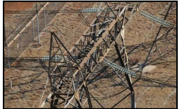
Fig. 12 An aerial inspection photo taken by Eskom.
