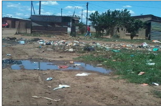
Plate 6.1: Subserviced roads, uncollected refuse and informal backyard dwellings
