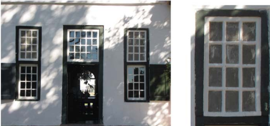
Figure 11: The fake upper lights of the half-width windows (Photograph: M. Burden, 2010)
