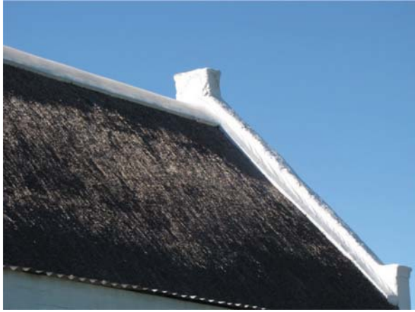
Figure 9: Chimney end-gable of manor house, 2010 (Photograph: M. Burden, 2010)
