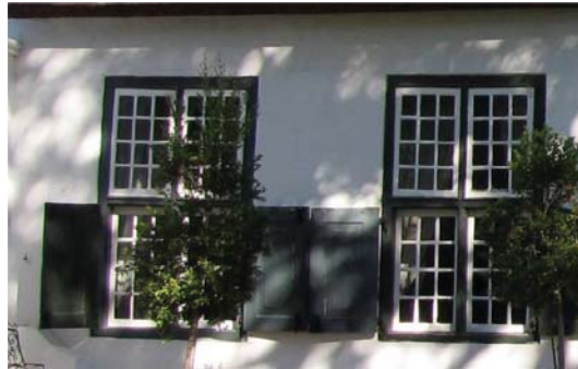
Figure 10: The cross-effect of the fixed upper- and casement lower-windows on the façade of Matjieskuil manor house (Photograph: M. Burden, 2010)
