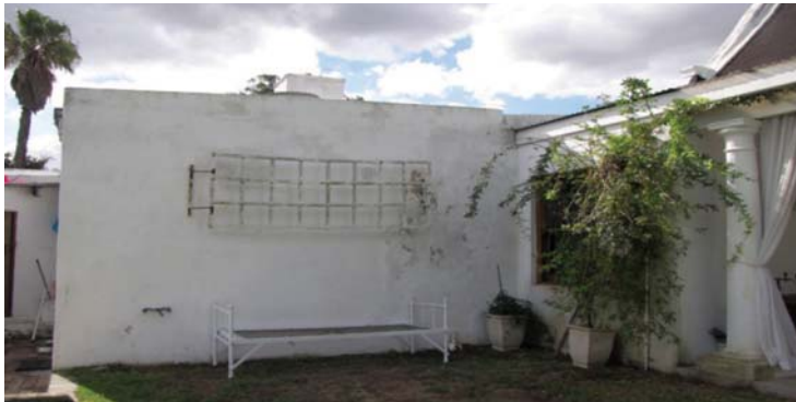
Figure 14: “Soutkamer” in its present form, flat-roofed and attached to the house, 2011
