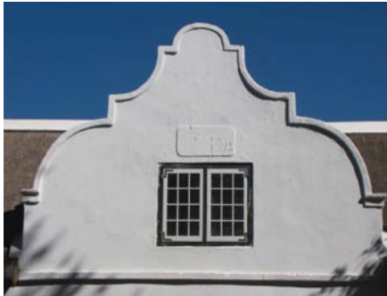
Figure 6: Front-gable of Matjieskuil manor house
