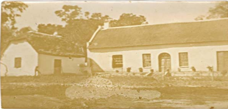
Figure 13: Back of the house, showing the loose standing thatched roof “soutkamer” (date unknown)
