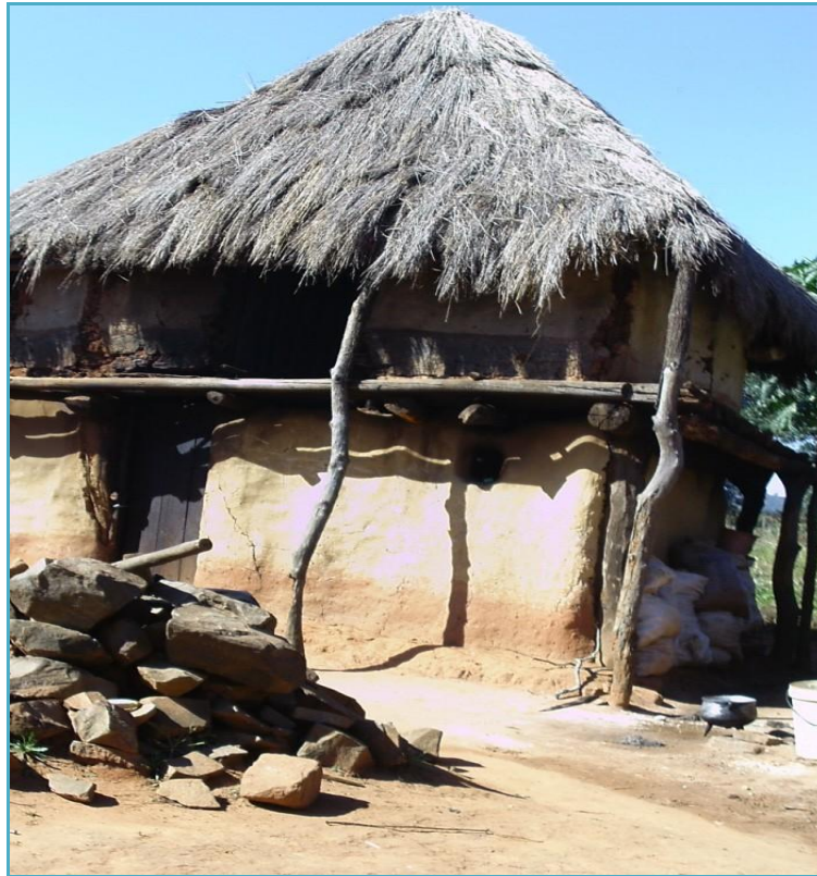
Figure 7.3 Double storeys Kitchen with upper part for seed preservation (Source: Researcher's personal photo library)
