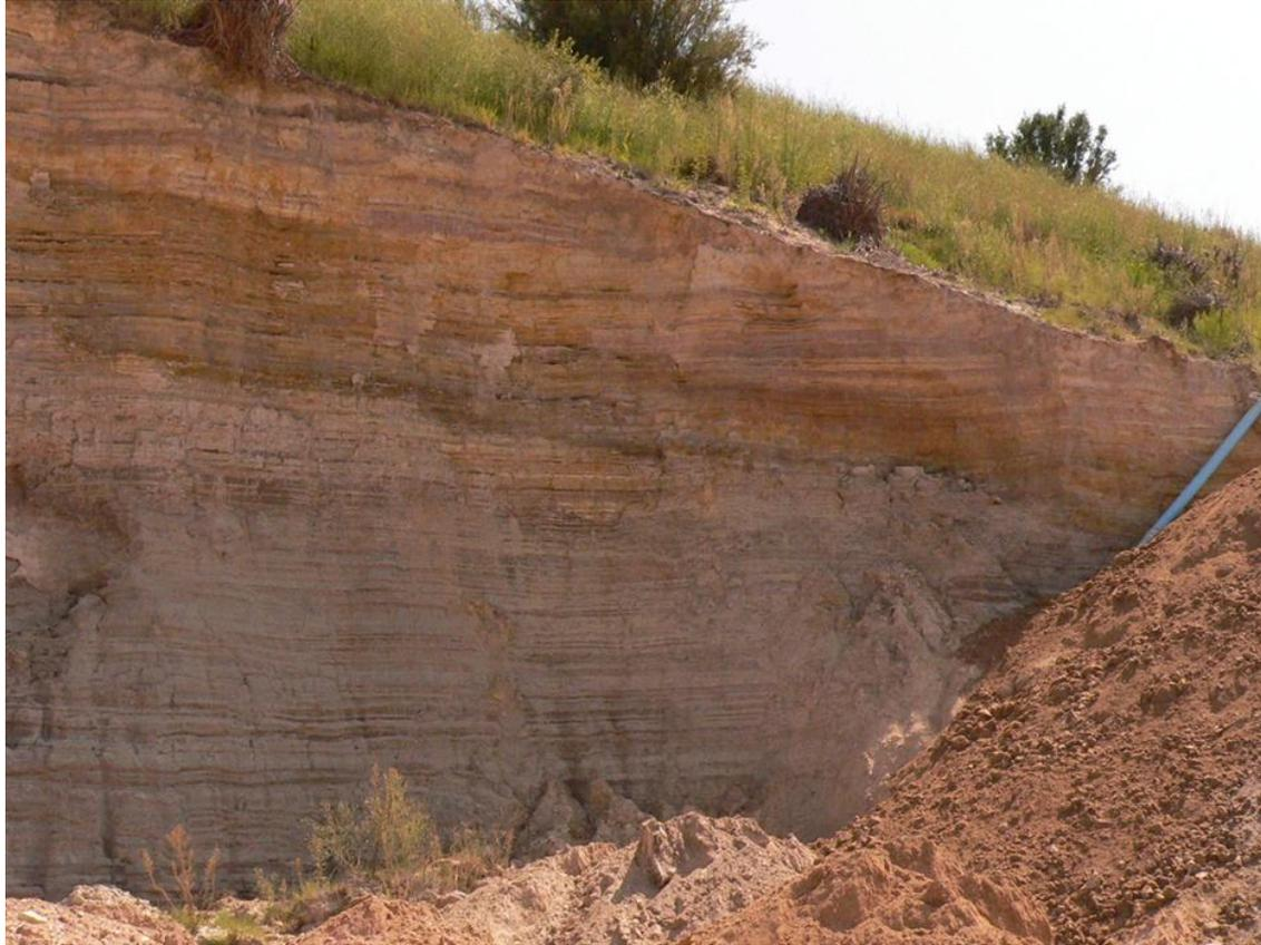
**Photo 2.1: Typical hydraulic separation layering in gold TDFs (Photo by P.W. van Deventer)**
