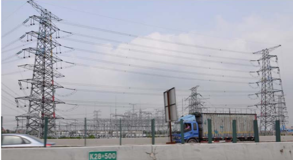
Figure 116: Multi-circuit lines
