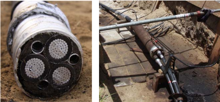
Figure 107: 66 kV oil-filled cable repair - joint bay
