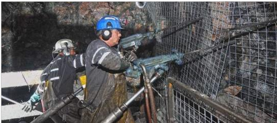
Figure 1-11: Pneumatic rock drill 3
