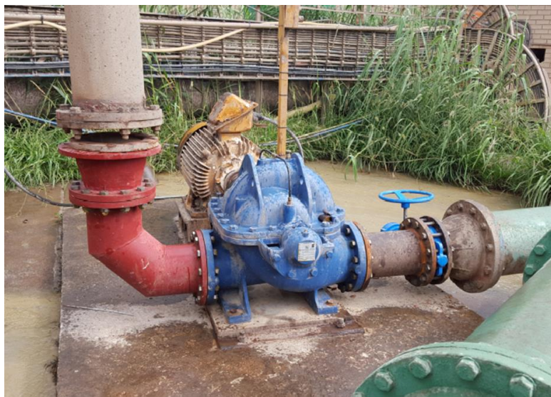
Figure 47 - Additional pump installation
