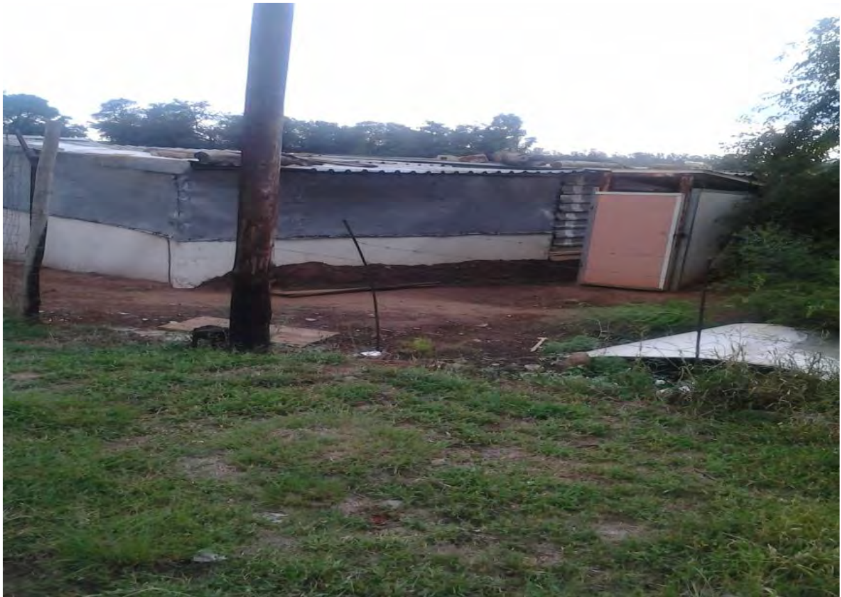
Photo 29: A pit latrine facing south ward of the dwelling (Photo: M. Mokoena, 2015)
