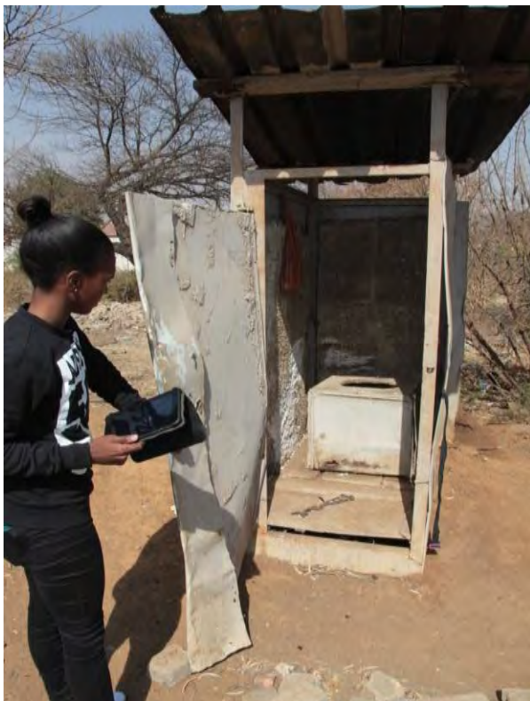
Photo 38: The plastic bag inside the latrine of the informal shop containing sawdust. That is sprinkled over the faeces after each toilet use (Photo: J.W.N. Tempelhoff, 2015)
