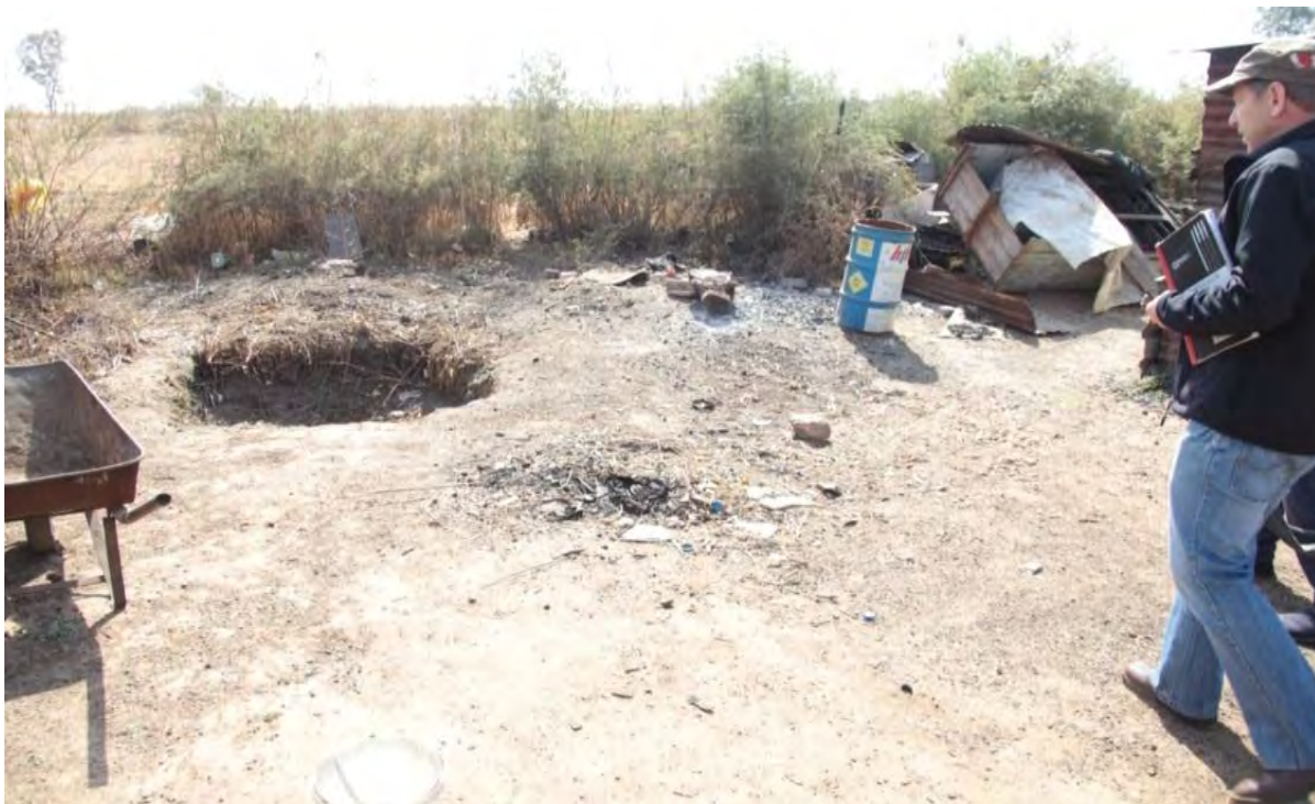
Photo 26: Pit latrine under construction in Mr Abiel Senooe's yard (Source: J.W.N. Tempelhoff, 2015)
