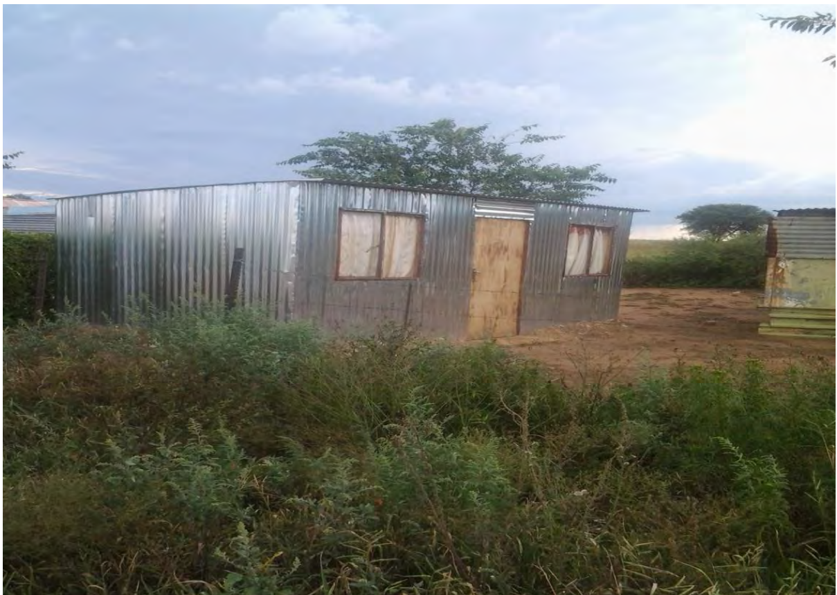
Photo 9: Typical two room zozo in BIS with ventilation (Source: M. Mokoena, 2015)
